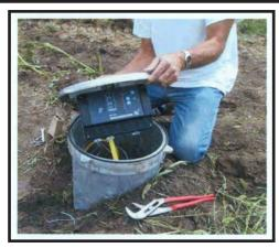
Controls mounted on plate attached to lid
